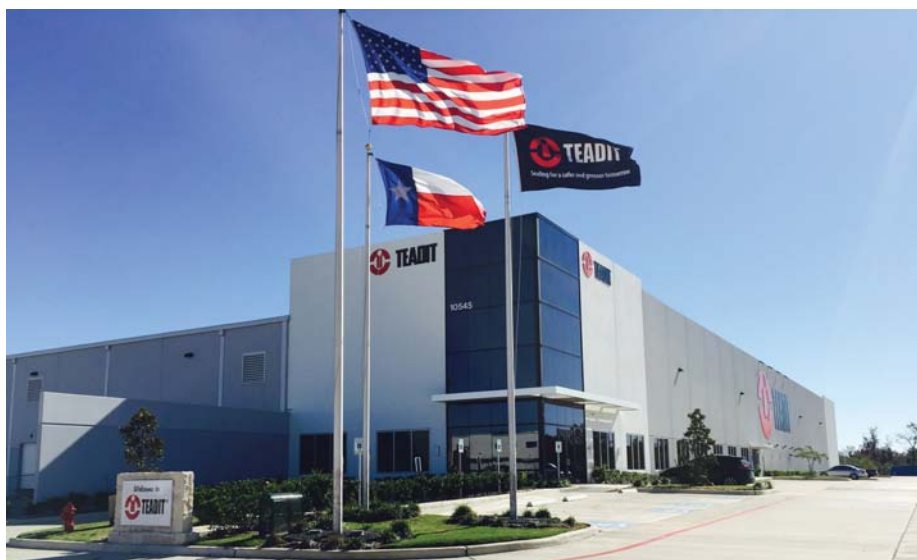
TEADIT manufacturing facility, Texas, United States.
