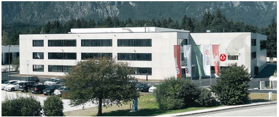
TEADIT manufacturing facility, Kirchbichl, Austria.
